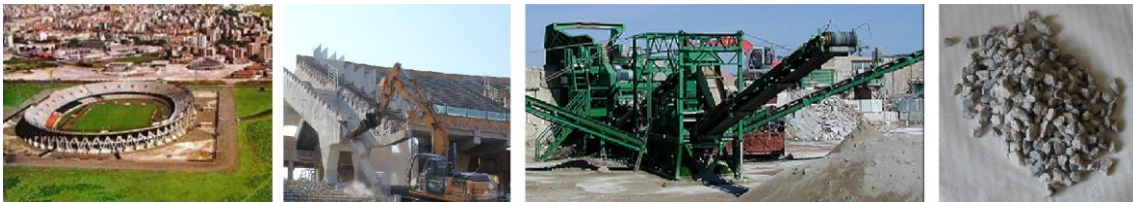
Figure 1. By demolition to production of RA
